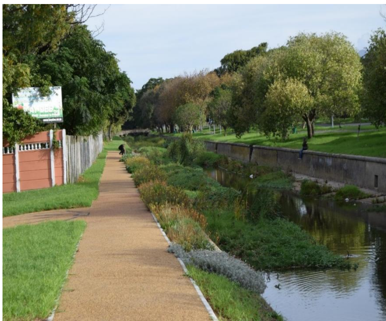
Figure 5. The pathway installed along Liesbeek River. Extracted from: Winter (2018a).
